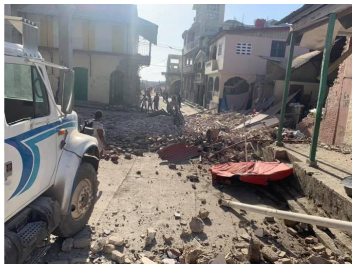
Damage to Downtown Jérémie
